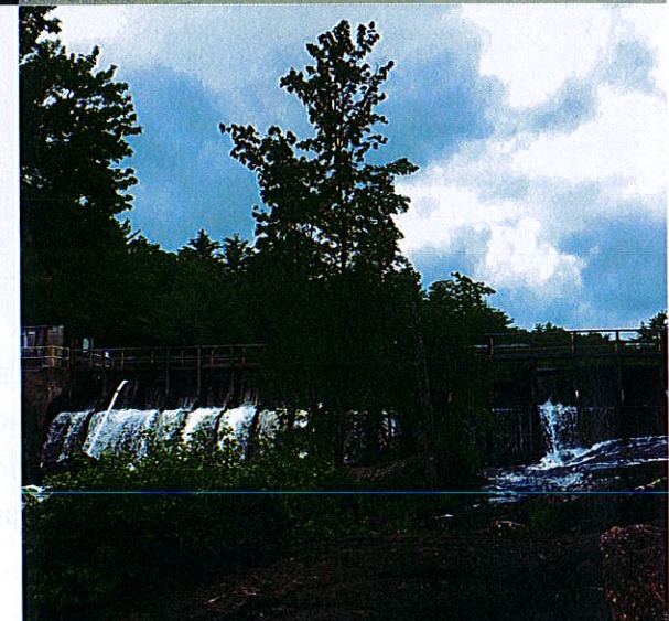
SFR Hydro, Milton
