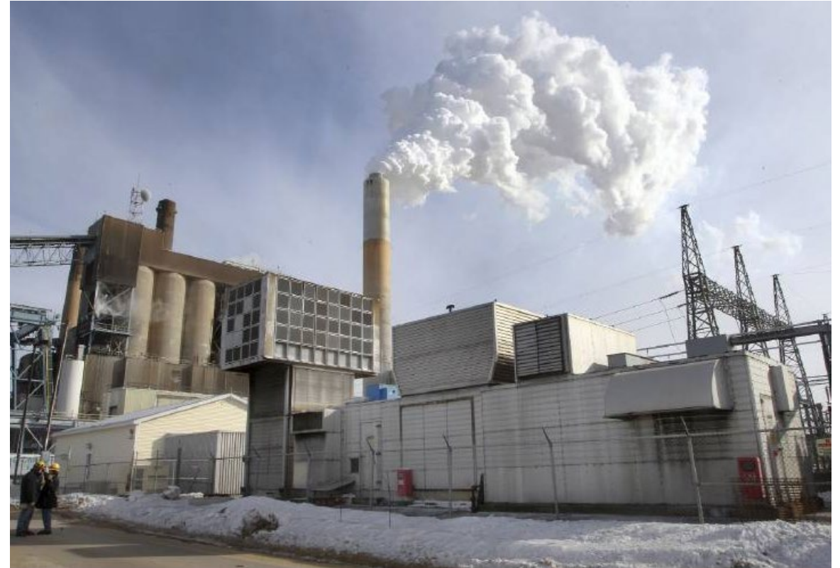
Merrimack Station in Bow, N.H., in 2014. Jim Cole/AP
